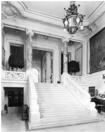
BELOW (counterclockwise): The yacht club's main staircase, library and lounge from archive photos of its opening in 1901.
